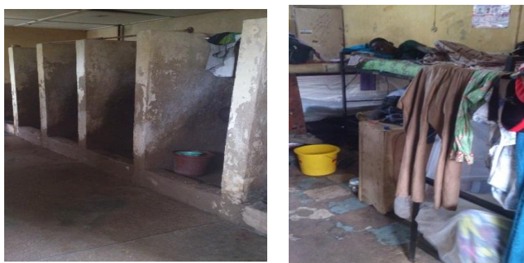
Plate 2: The present conditions of room, toilet and bathroom within students' hall of resident in OAU Source: field survey, 2015
